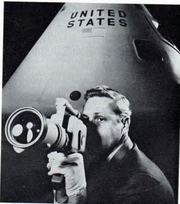
Original hand-held TV camera developed for the Apollo programme.
