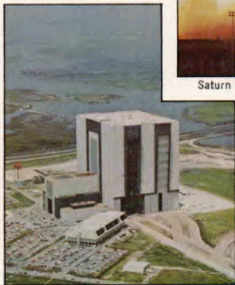
Vehicle Assembly Building
