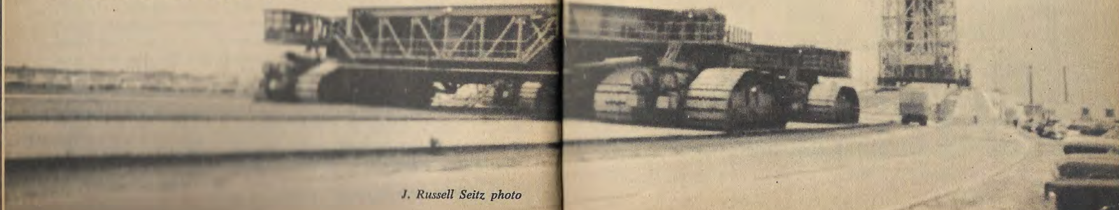
The crawler en route to pick up another few kilotons of equipment.
